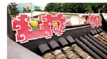
The plastered reliefs of Kuilong at the ends of the ridge 屋脊兩端的夔龍的灰塑
