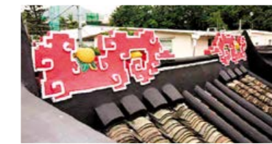
The plastered reliefs of Kuilong at the ends of the ridge 屋脊兩端的夔龍的灰塑
